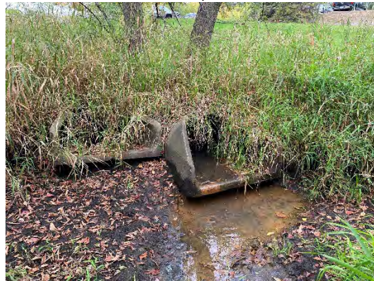
Photo 4: Culvert outfalls Reach 16
