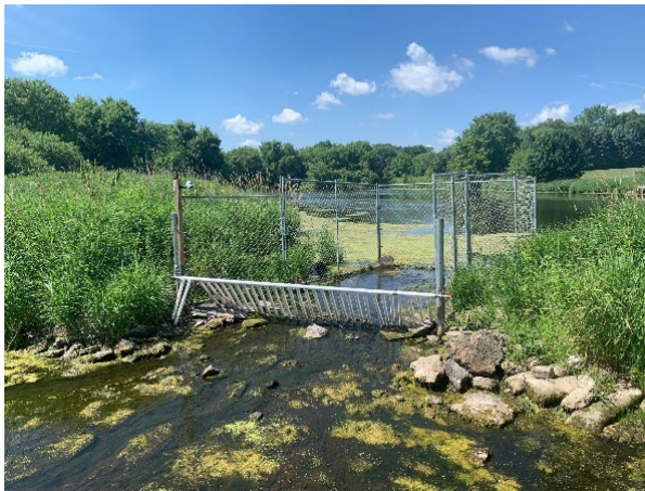
FIGURE 7: NOVEL CONCEPT KNOWN AS A PUSH TRAP INSTALLED IN A STREAM.
