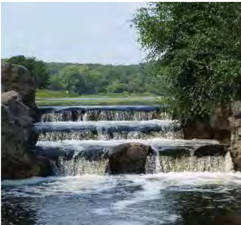
Normandale Lake features a natural-appearing boulder outlet structure.
