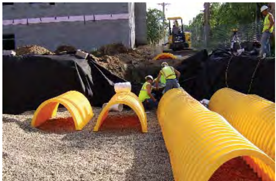
Infiltration pipes being installed under a parking lot near Glen Lake.
