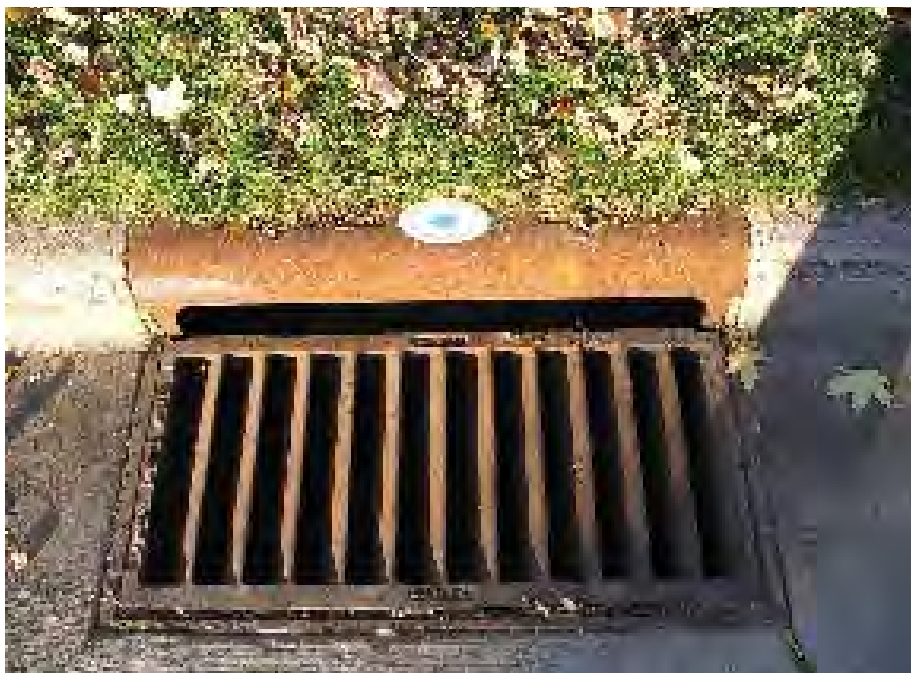
Storm drains in the NMCWD are labeled with "no dumping" signs, reminding residents that local stormwater reaches Nine Mile Creek.
