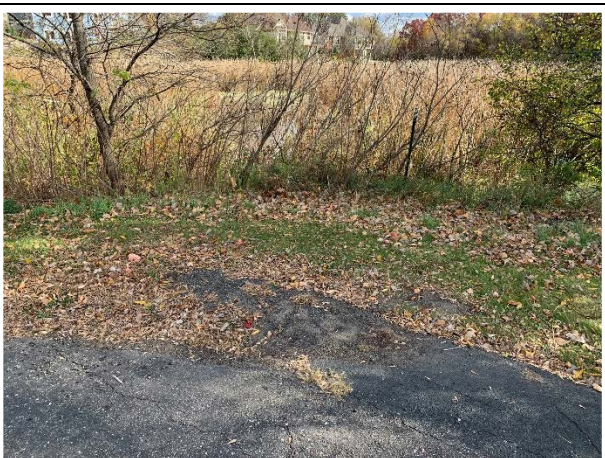
Wetland 27-116-22-02-027 – sediment directed into wetland
