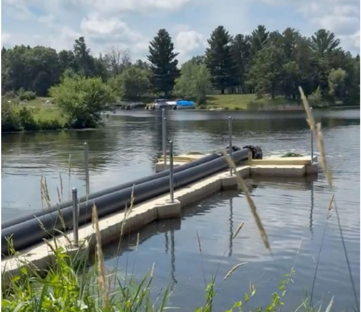
Figure 7-3 Moleaer nanobubble feed pipes
