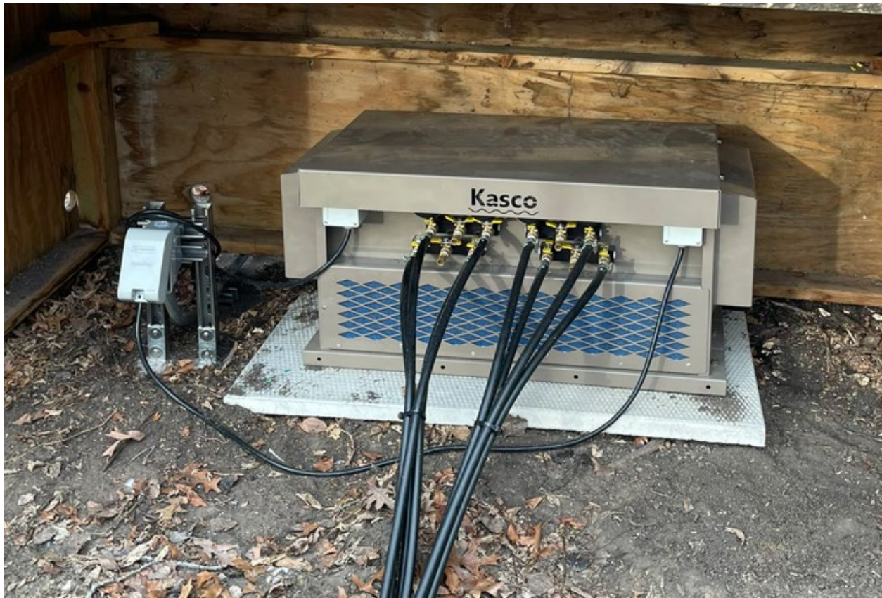
Figure 7-1 Typical aeration enclosure for diffused-air aeration
