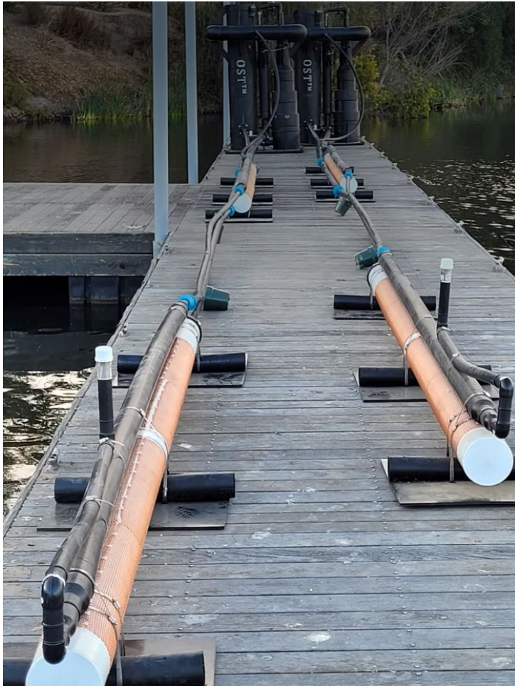
Figure 7-5 OST system on shore prior to deployment
