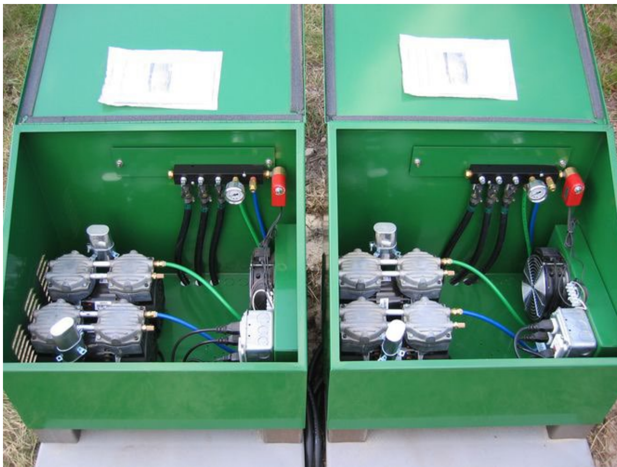
Figure 7-2 Aeration compressors for diffused-air aeration
