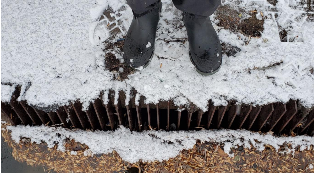
Figure 6: A grate covers the culvert where water runs to North Cornelia Lake. It is unlikely that adult or subadult carp could pass, but possibly small goldfish.
