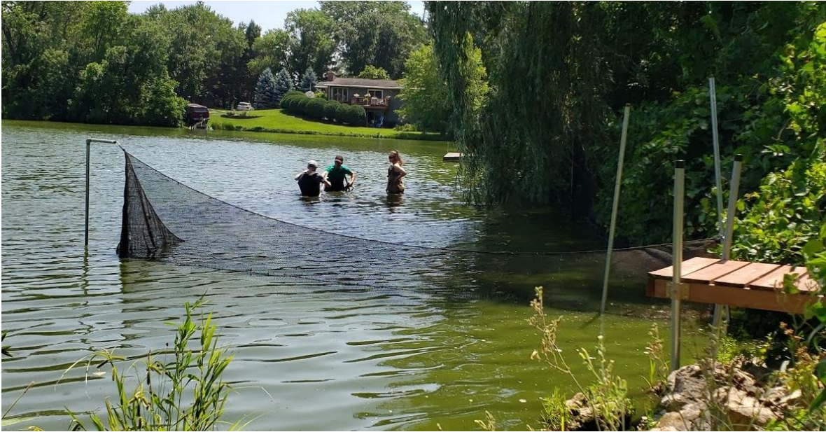
Figure 9: In the process of installation of the box net in the Northwest corner of Lake Nancy.
