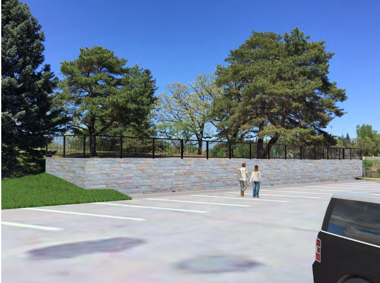
Figure 4-5 Rendering showing the approximate size and location of the concrete filtration vault with limestone facing on vault walls
