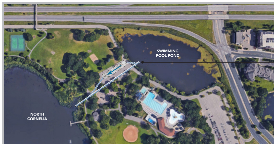
Water moves through the spent lime filtration chamber to remove phosphorus before discharge to Lake Cornelia.
