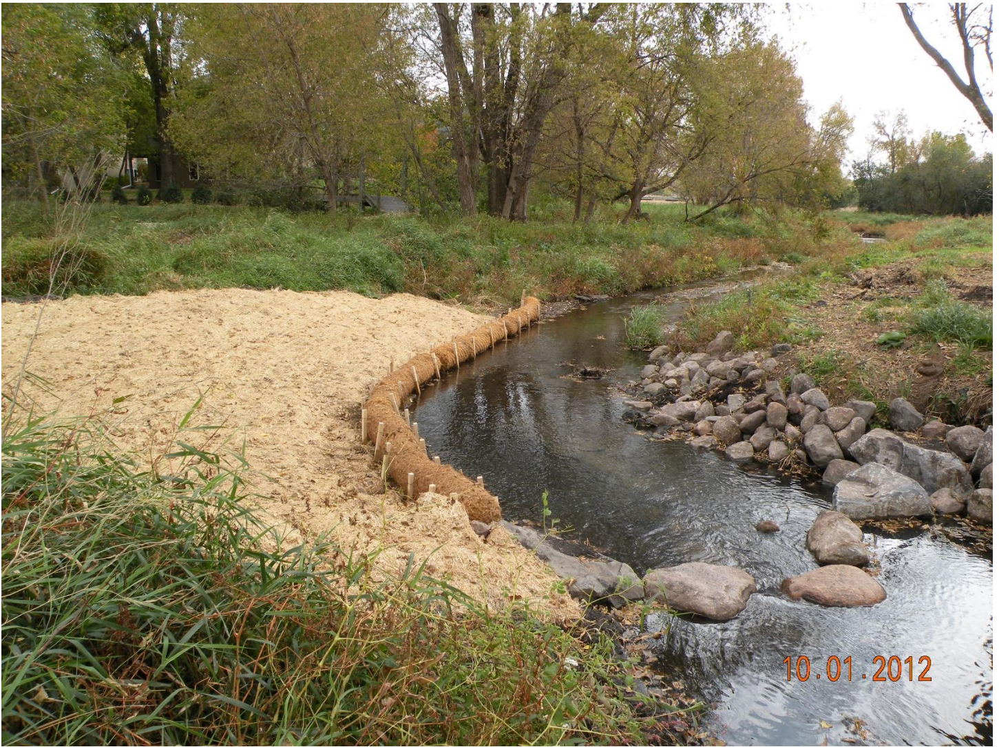
Rock riffle at a site in the City Hopkins portion of the project.
