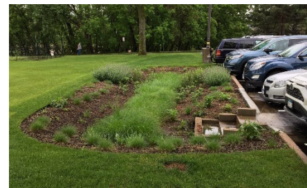
Raingarden during inspection
