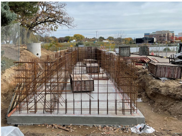
Installing rebar for the vault walls to prepare for pouring concrete.
