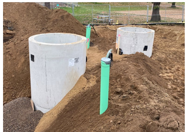
Pump and metering manholes installed
