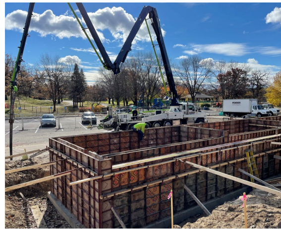
Wall framing and concrete pouring of vault walls
