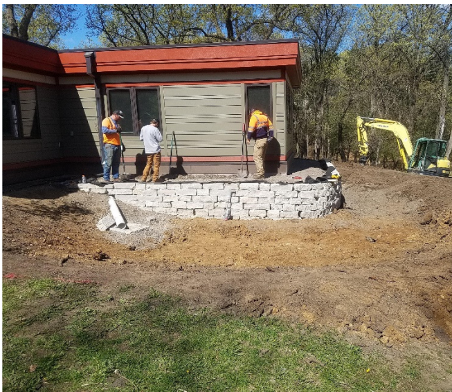
Left: The maintenance strip above the rain garden is being constructed. Loosened soils in the foreground will be good for infiltration. Right: A lone nodding trillium flower blooms in the newly cleared and seeded restored area
