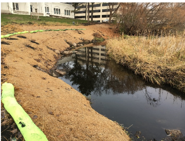
Rock vanes providing bank protection in Reach 14
