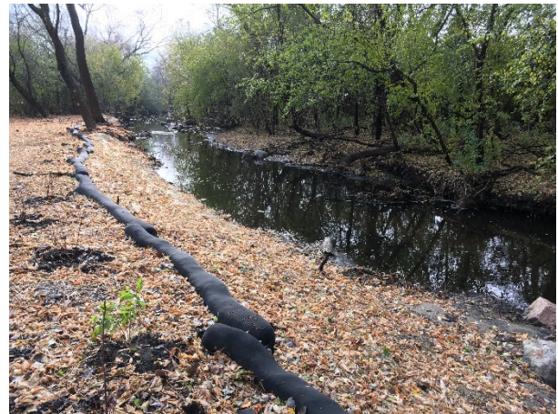
Graded banks with log vanes in Reach 13.
