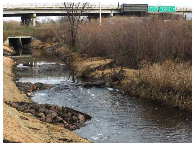
Reach 15 graded banks, cross vane, and outlet protection
