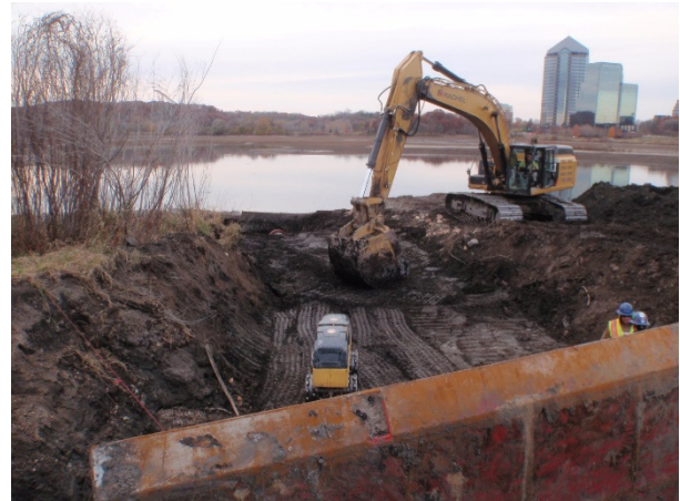
Installation of upstream portion of 36-inch HDPE bypass pipe.
