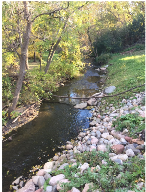
Graded banks with rock vanes, riprap, and new vegetation in Reach 10 (Phase I).
