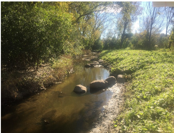
Rock vanes and new vegetation in Reach 6 (Phase I).
