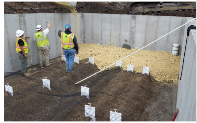
Photos show construction of an underground spent lime filtration BMP in the Ramsey-Washington Metro Watershed District.
