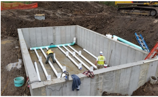
Photos show construction of an underground spent lime filtration BMP in the Ramsey-Washington Metro Watershed District.
