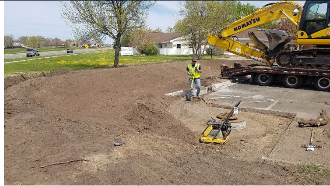
Final grading of the planting soils and adjustment of the overflow structure at St. Luke's Church in Bloomington.
