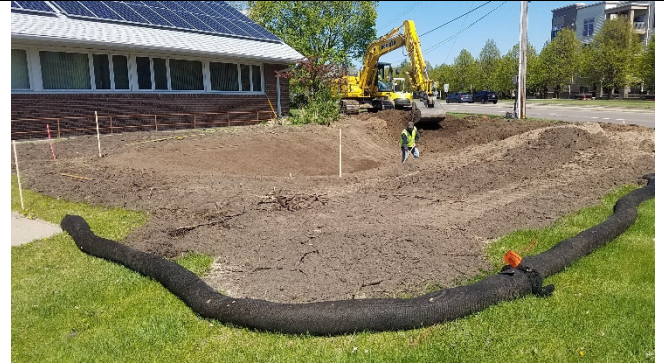
On the busy corner of Old Shakopee Road and Penn Avenue in Bloomington, Sunram Construction measures planned depths of the rain garden.
