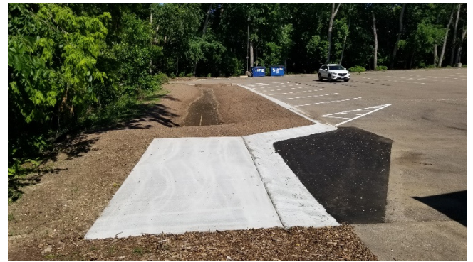
Splash block assembly, curb and pavement installation completed at Good Samaritan Church in Edina, ready for planting.
