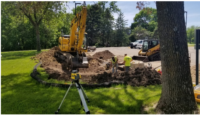
Excavation, placing planting soil, and preparation for splash block installation for raingarden #1 at St. Edward's Church in Bloomington.
