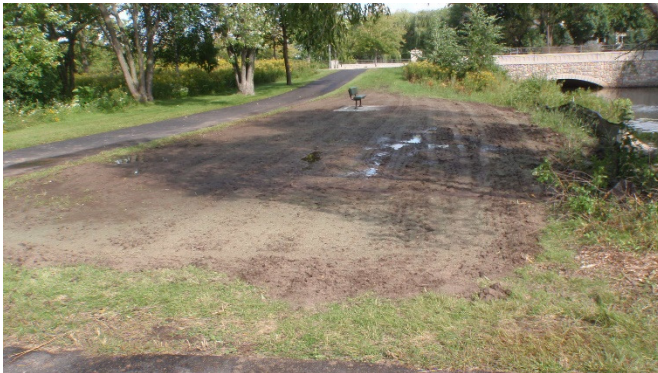
Photo of restoration area at the creek inlet on the north side of Normandale Lake. A contractor hired by the City of Bloomington recently installed a memorial park bench in the area disturbed and partially restored by Rachel Contracting as part of installation/removal of the temporary weir in the creek channel (photo from September 10, 2019). The City of Bloomington will complete the restoration efforts in this area.
