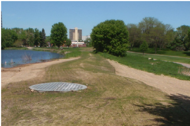
Restoration of disturbed areas at bypass pipe and manhole location (photo taken May 28, 2019).
