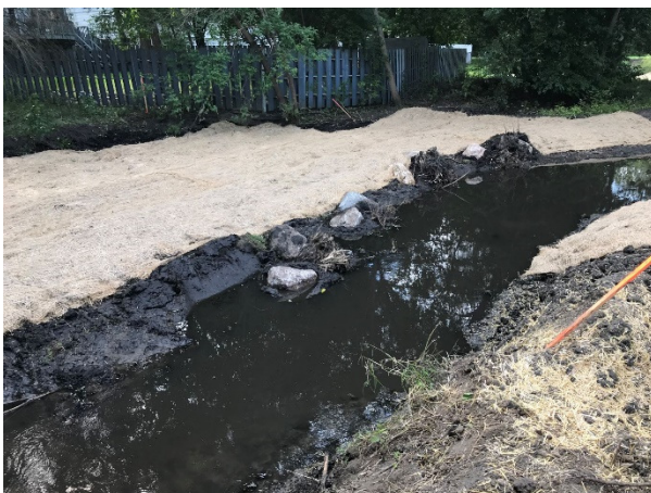
Phase 2 stream remeander with root wads.
