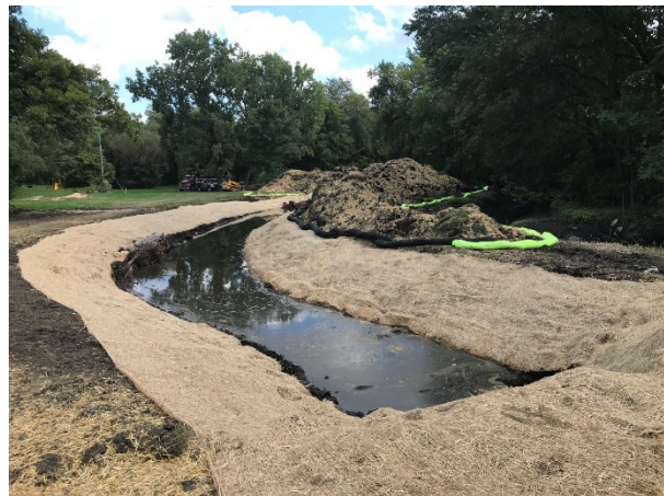
Phase 2 stream remeander with rootwads.
