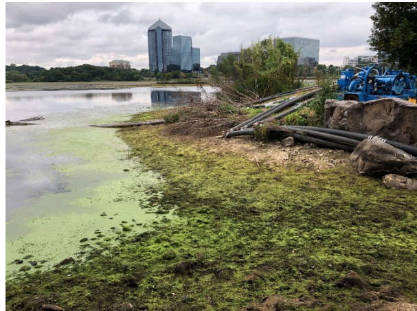
Exposed lake bottom at lake outlet structure.
