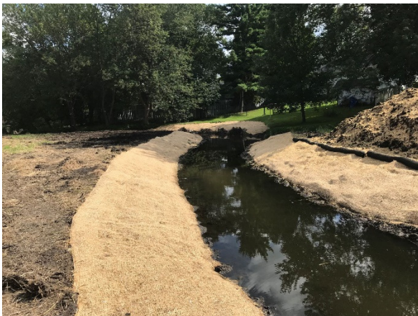
Phase 2 excavated and seeded stream remeander.
