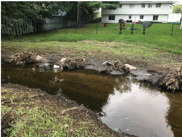
Phase 2 stream remeander with root wads held up to flood flows.
