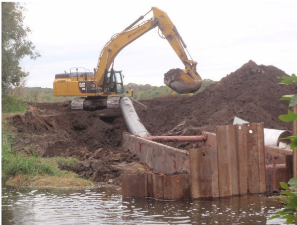
Installation of downstream portion of 36-inch HDPE bypass pipe, which discharges into Nine Mile Creek downstream of the Normandale Lake outlet structure.
