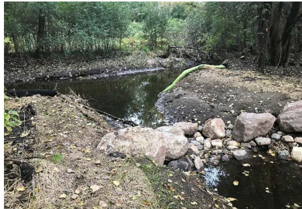
Phase 2 rock vane at the entrance channel to off-channel pond.
