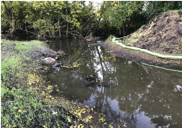
Phase 2 grass growing in excavated channel after flood.
