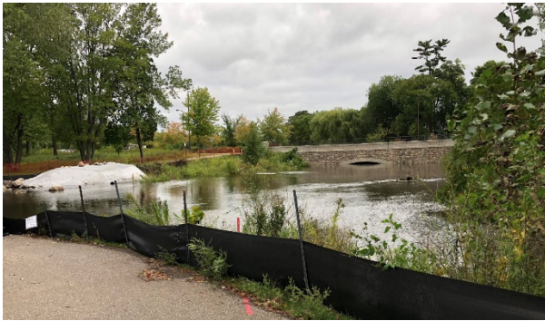
High water levels in upstream channel after 3-inch rain.
