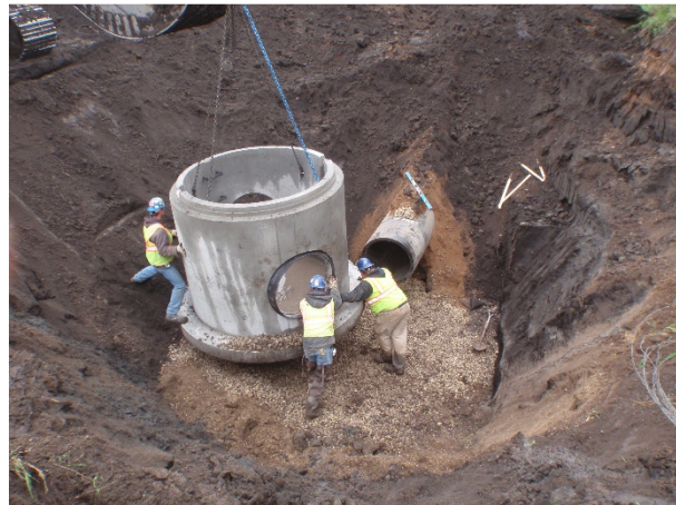
Installation of manhole structure on the 36-inch bypass system. Stop logs will be installed inside the structure to prevent passage of water and refill the lake in spring.
