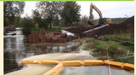
Floating silt curtain that protects lakes during construction
