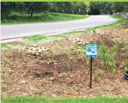
New rain garden with Nine Mile Creek Watershed District sign
