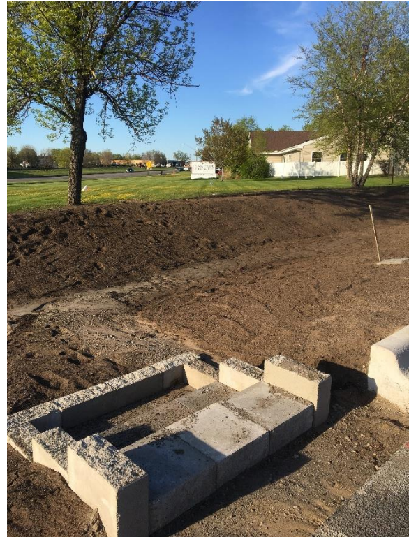
Raingarden Basin During Construction, 2020
