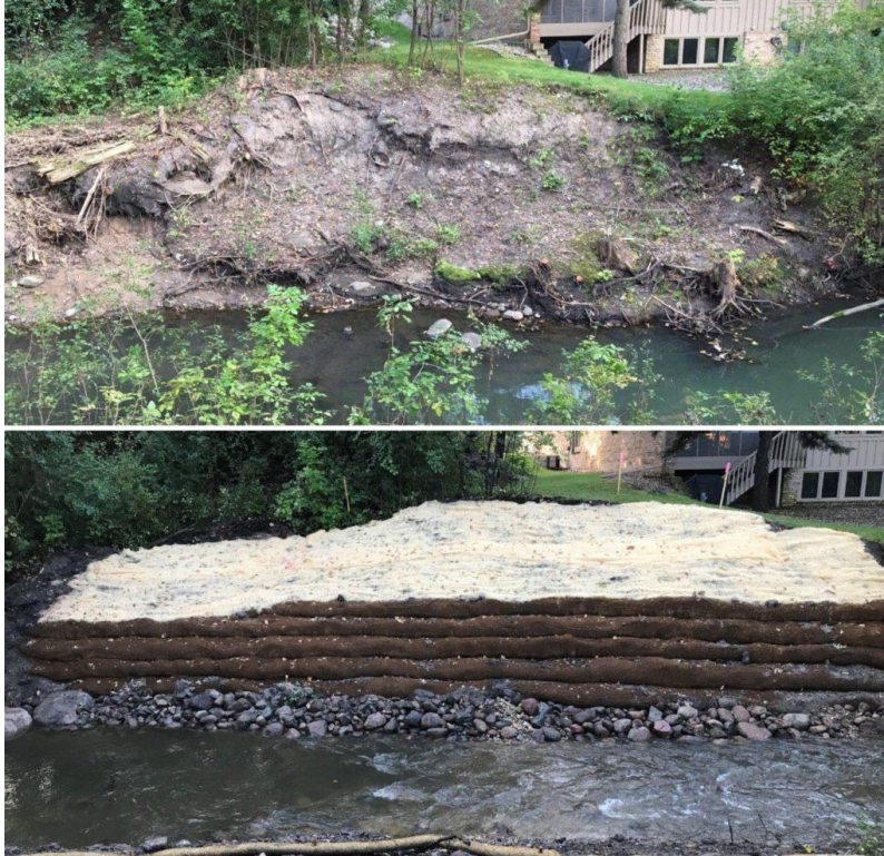
Before and during restoration – vegetative reinforced slope stabilization
