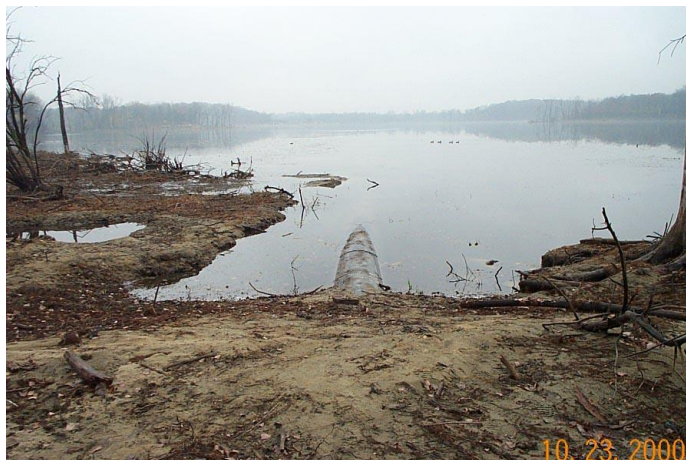
Newly installed outlet pipe; 2000. Notice flood impacted vegetation.
