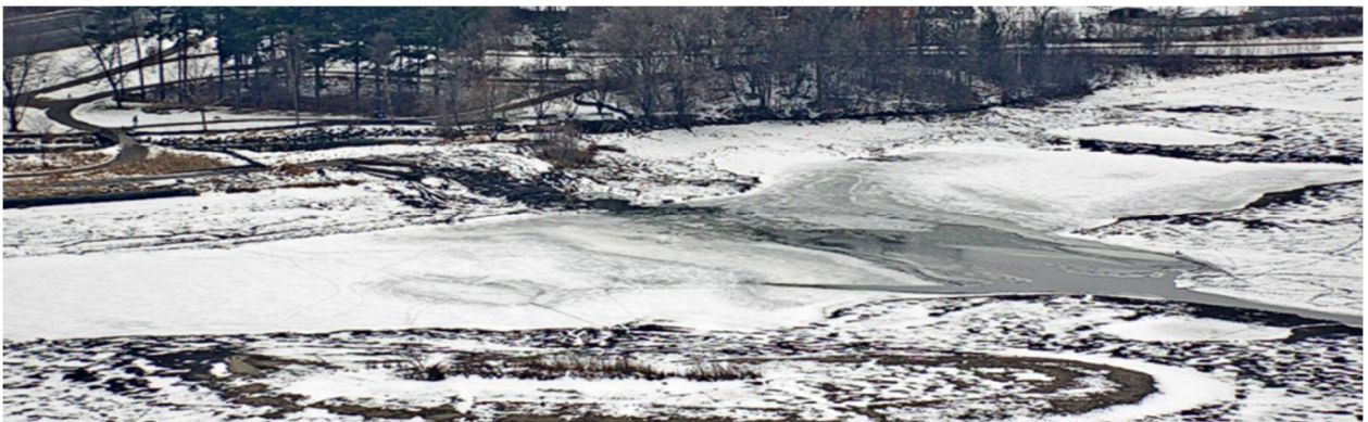
Photo following deployment of deicer system at the upstream edge of the ice bridge covering the main channel. City staff reported that after about 90 minutes of operation, the deicing system had opened up a 10-foot span area of water.
