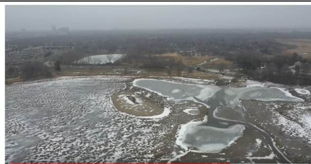
Aerial view of remaining standing water during drawdown (ice covered) near outlet of Normandale Lake (December 22, 2018).
