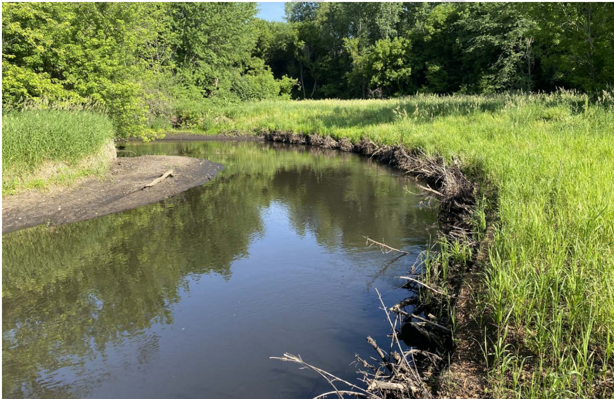
Figure 11. Example of Toewood Installed Post-Construction
