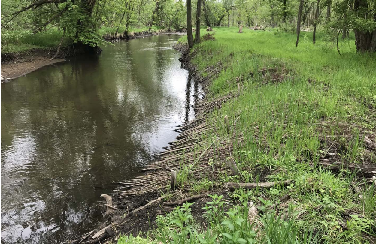
Figure 12. Example of Brush & Rootwads Installed Post Construction
