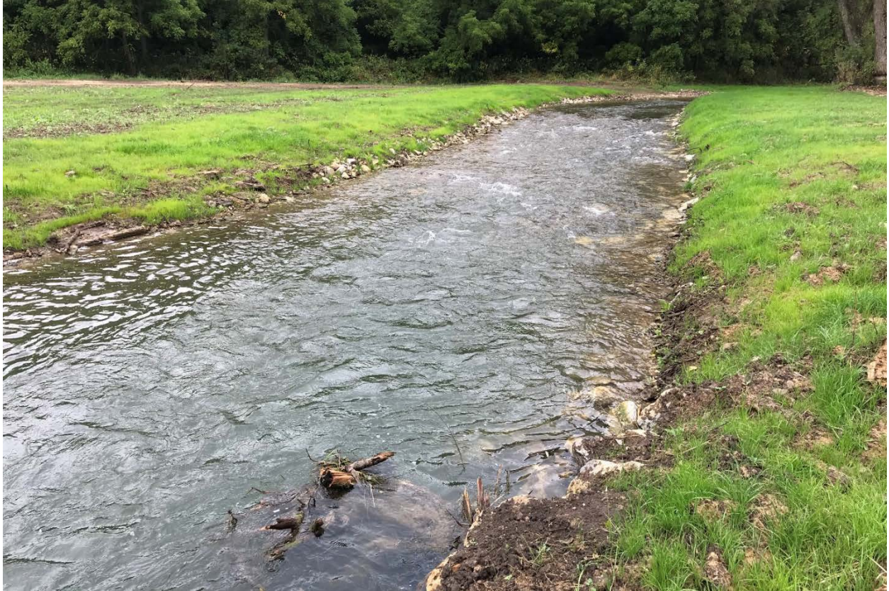
Figure 13. Example of Riffle Grade Control and Deep Pool Habitat with Rootwads
