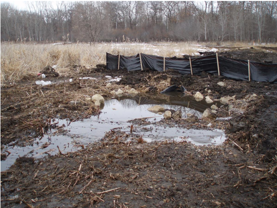
Photo 5: Birch Island Inlet during Construction showing riprap (2007)
