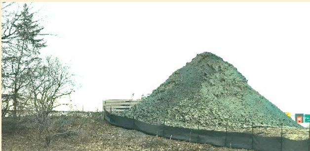
Above: Hydromulch sprayed on top of stockpile
