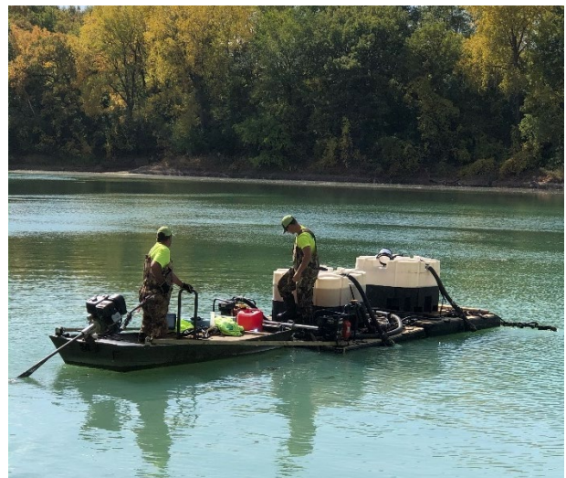
Figure 4-2 Examples of treatment barges that may be used to apply ferric chloride and sodium aluminate to Arrowhead Lake
