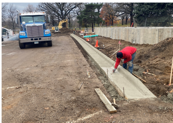
Curb and gutter installation
