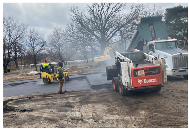
Bituminous pavement installation
