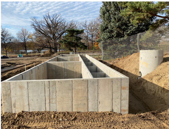
Concrete walls for filtration vault completed
