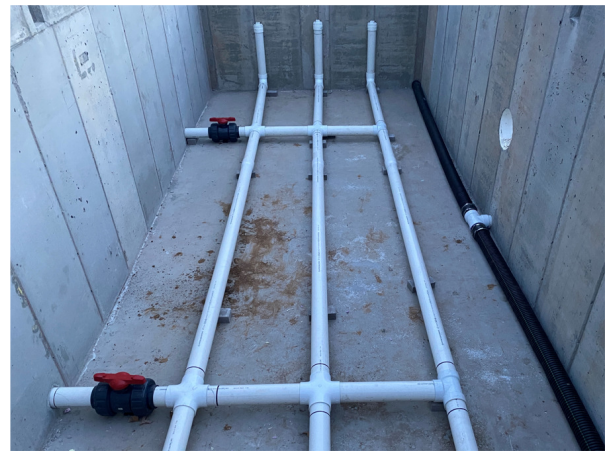
Filtration vault drainfile installation
