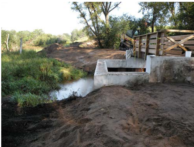
The hydrology for an existing wetland was restored by constructing a new outlet structure
