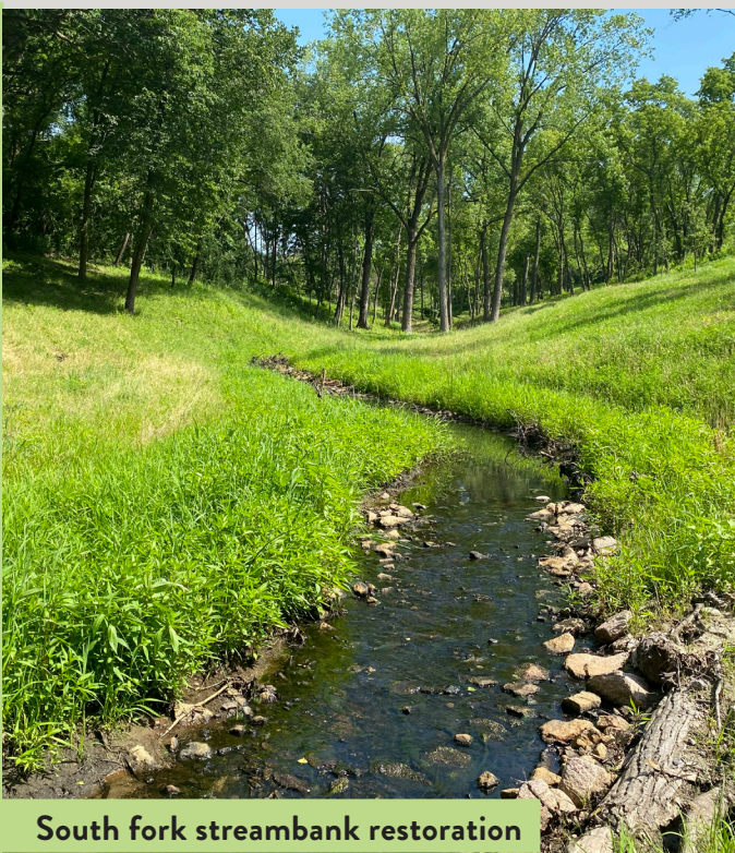
South fork streambank restoration
