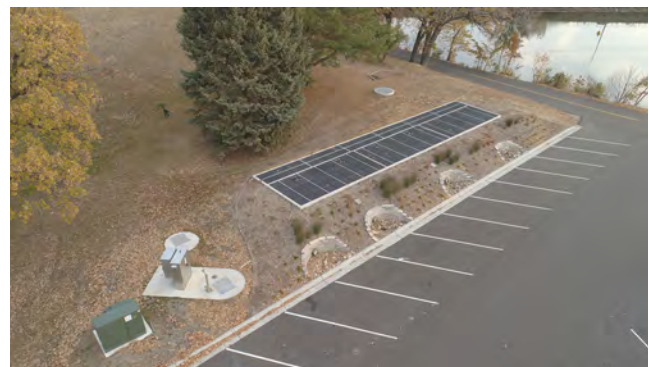
Rosland Park Stormwater Filtration Vault
