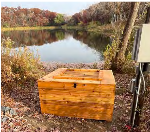
Aeration System Improvements
