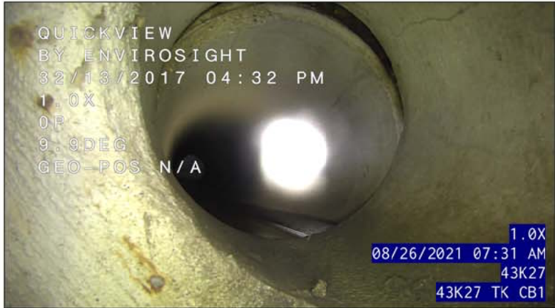
OFFSET JOINT AT FIRST JOINT FROM ST MH 11 TO ST CB 12
