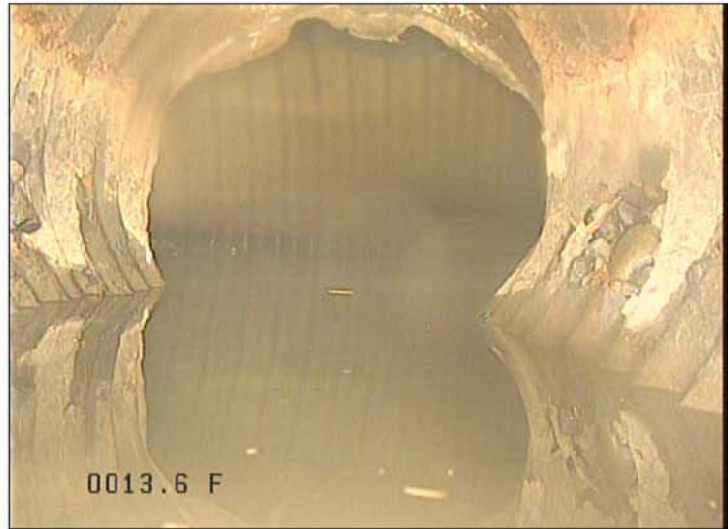
18" CMP CONNECTION AT 120" CMP
