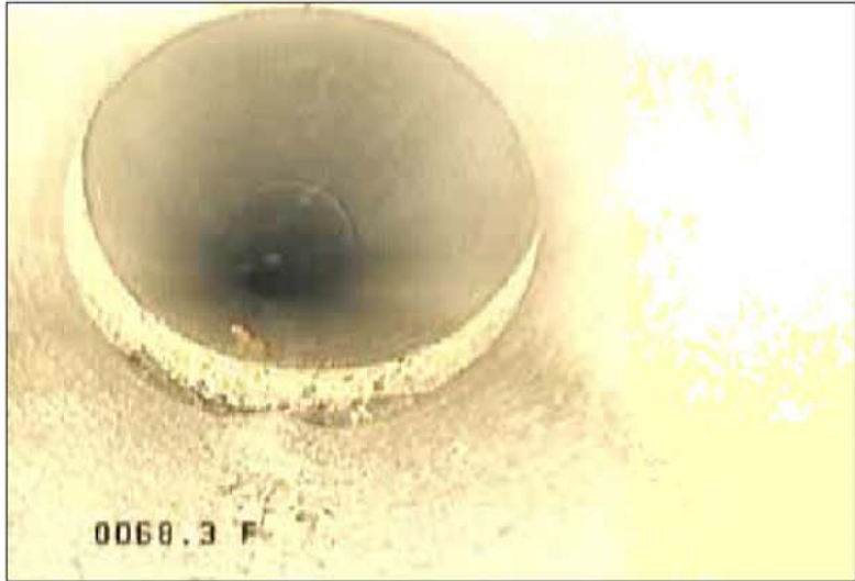
OFFSET JOINT APPROXIMATELY 71 LF FROM ST MH 11
