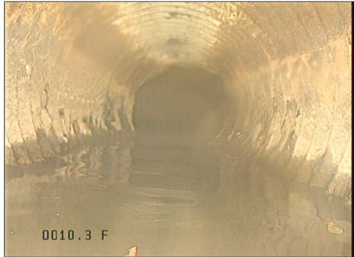
DETERIORATED 18" CMP
