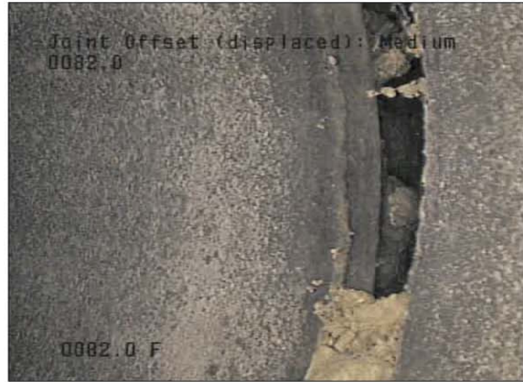
OPEN JOINT APPROXIMATELY 82' FROM ST MH 1
