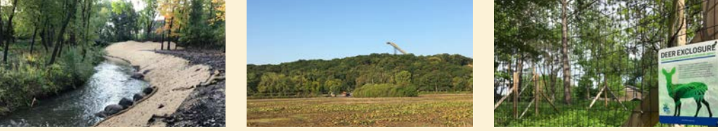
Left: Restoration work on Nine Mile Creek Middle: Normandale Lake drawdown Right: Deer enclosure structure in the restoration area
