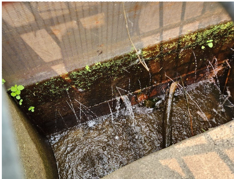
Figure 8-8 Photo of plugged Southeast Anderson macrophyte screen on top of stop logs (May 2025)
