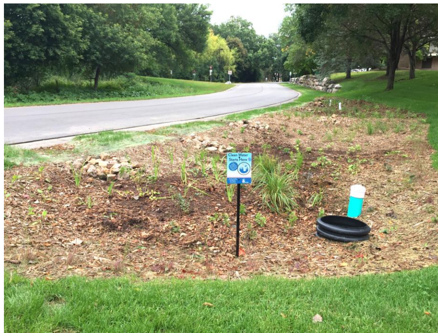
Raingarden installed at a condo association with a 2019 cost share grant
