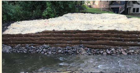
Before and After Restoration on Reach 1 of Nine Mile Creek
