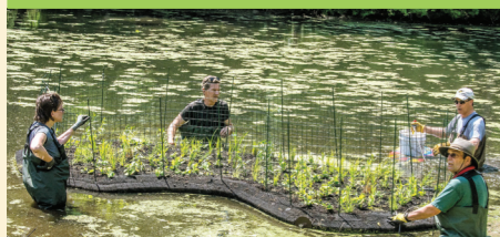
Floating Island Installed with a Cost Share Grant
