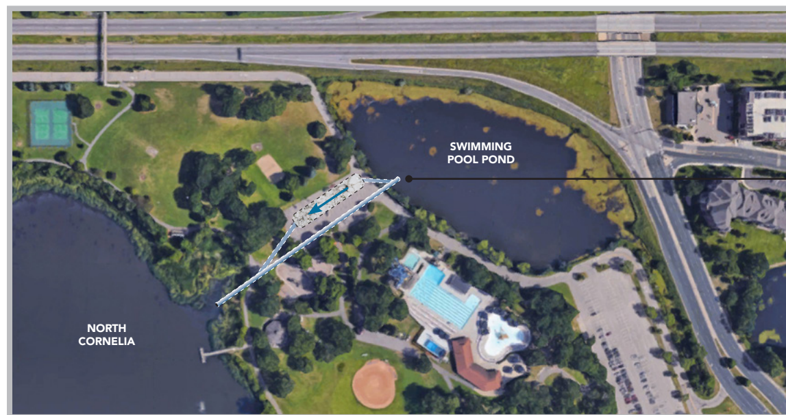
Water moves through the spent lime filtration chamber to remove phosphorus before discharge to Lake Cornelia.
