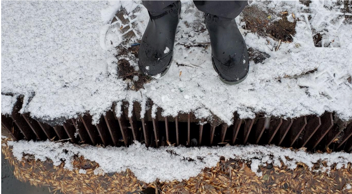
Figure 6: A grate covers the culvert where water runs to North Cornelia Lake. It is unlikely that adult or subadult carp could pass, but possibly small goldfish.
