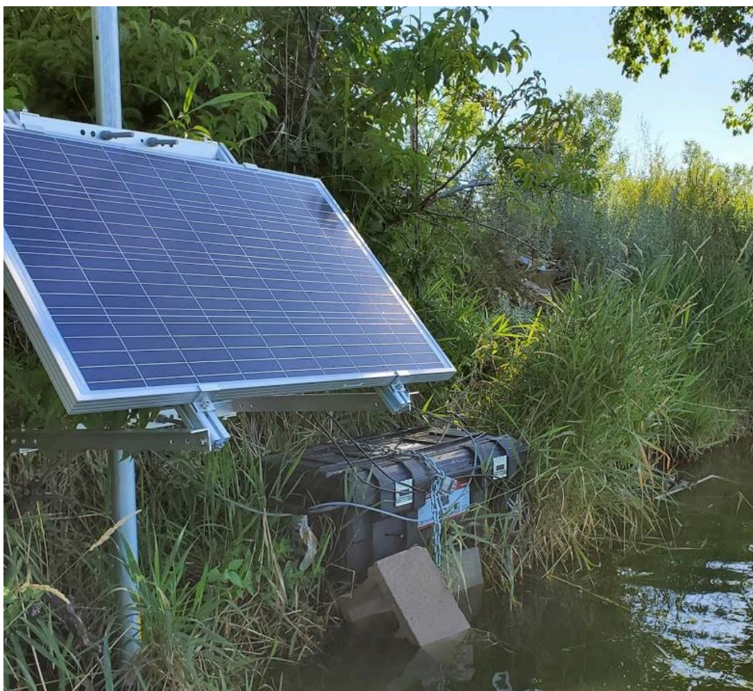
Figure 8: A solar powered PIT antenna station located between North and South Cornelia.
