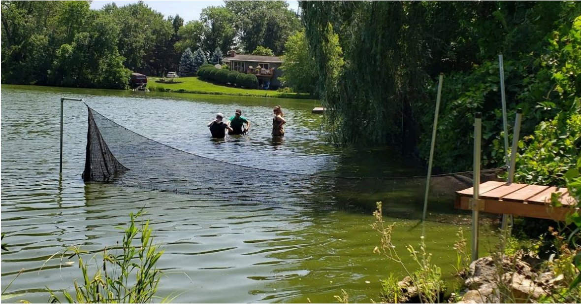
Figure 9: In the process of installation of the box net in the Northwest corner of Lake Nancy.
