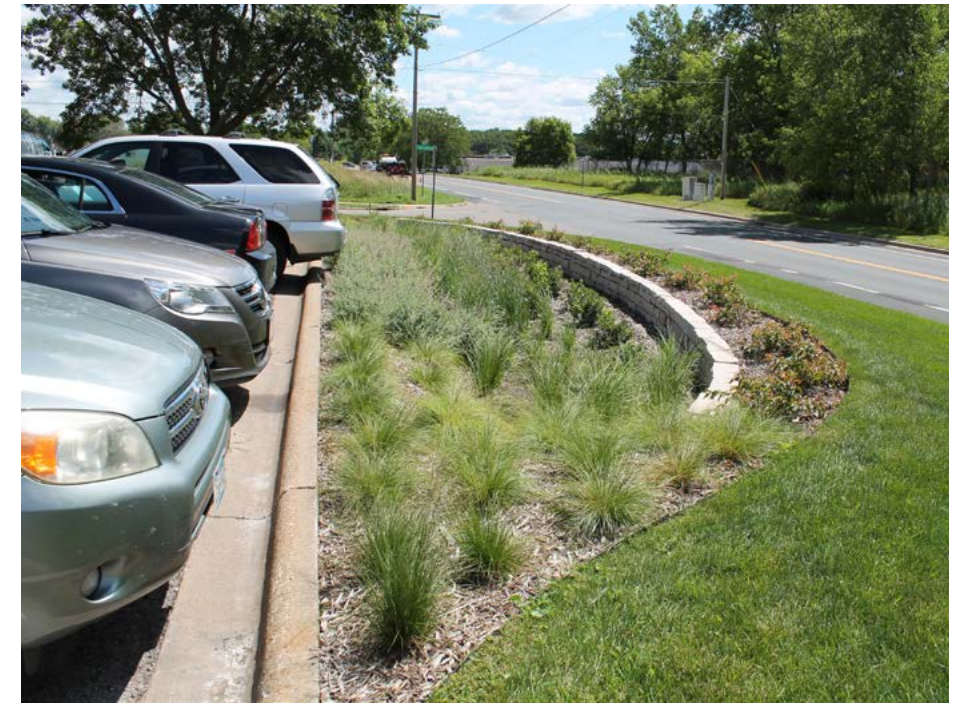
Swale (shallow depression that conveys water) with massings of ornamental grasses and shrubs.
