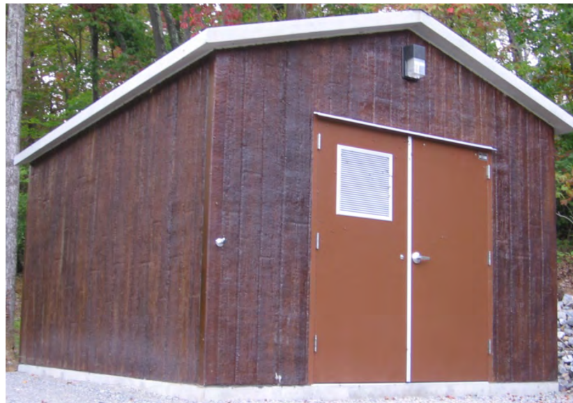
Figure 3.11: Example of a pre-cast building to house oxygen supply equipment
