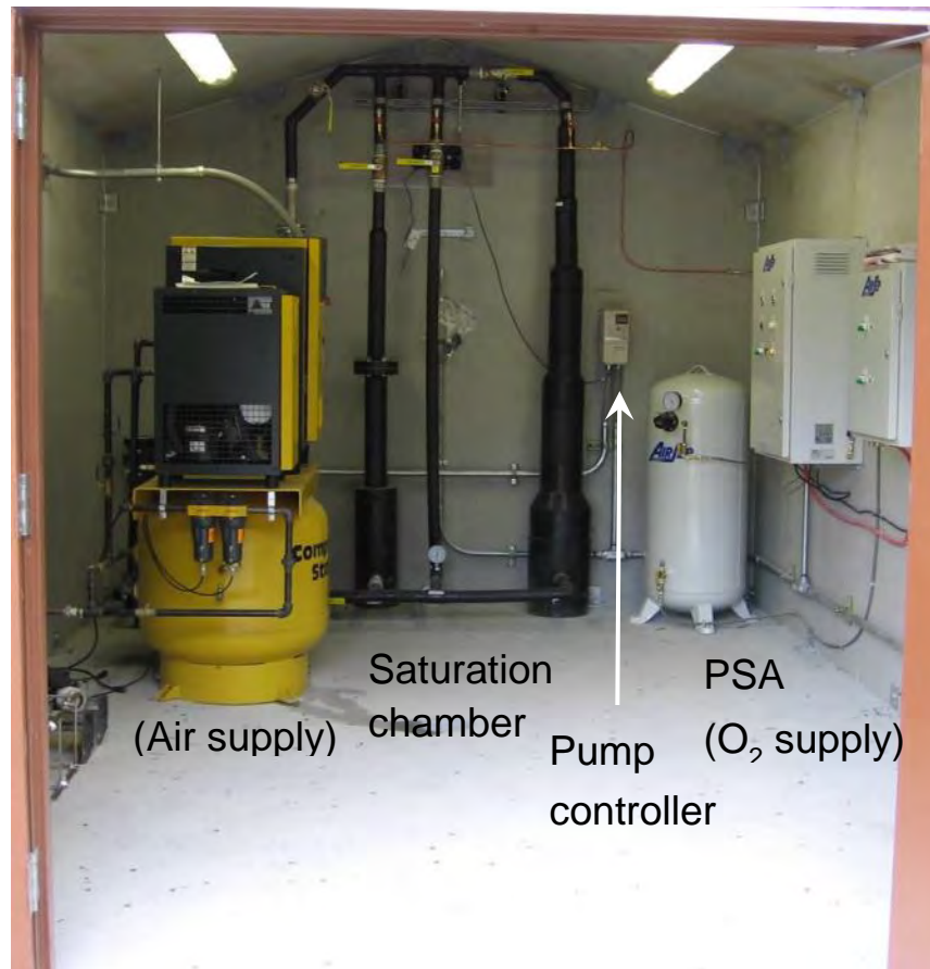
Figure 3.10: Photo of a precast concrete building used to house a Kaeser SX 7.5, a small Centrox oxygen generator and all piping for a small SSS oxygenation equipment.
