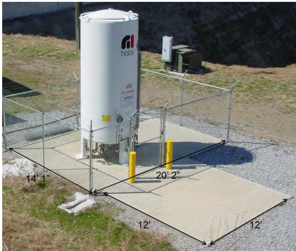
Figure 3.7: Example of a typical LOx system. Photo shows a 1500 gallon tank.
