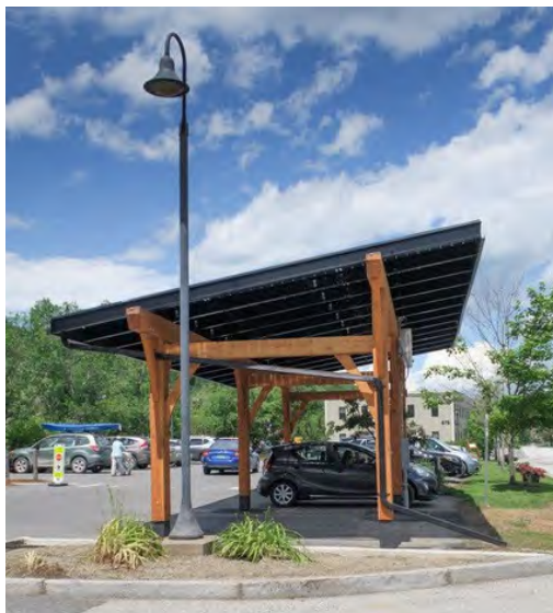
Image to the left: Timber frame and SunCommon's Solar Canopy.
