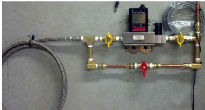
Figure 18: Example of Alicat flow control header with braided SS supply line from oxygen supply, brass fittings, and flexible copper out the outflow side to an oxygen contact chamber.
