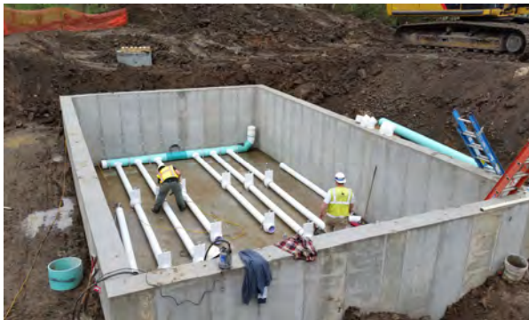
Ramsey-Washington Metro Watershed District Frost-Kennard Spent Lime Vault Filter
