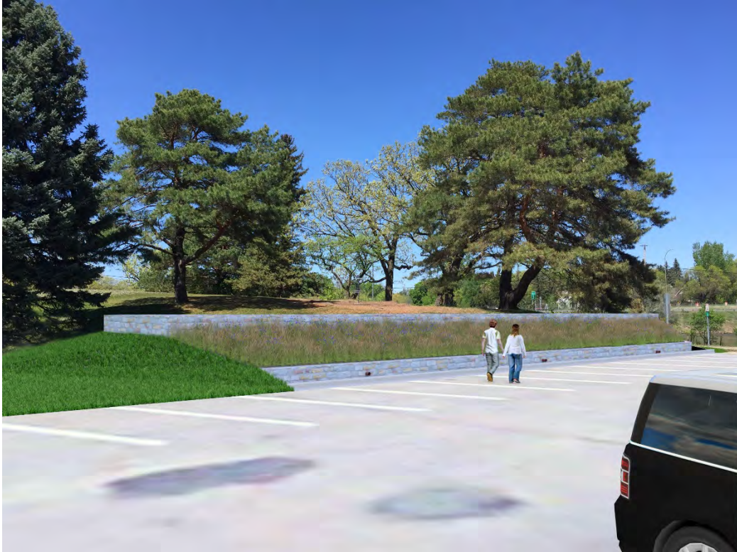
Figure 4-6 Rendering showing the concrete filtration vault with partially-buried vault walls and a low limestone wall
